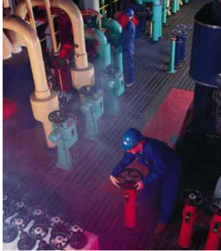
Charlottetown Thermal Generating Station
