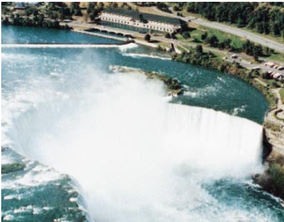
Aerial view of the Rankine Generating Station above Niagara Falls
