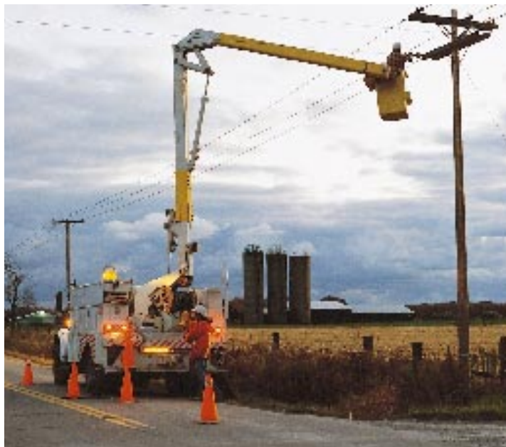
Utility operations are a Fortis strength
