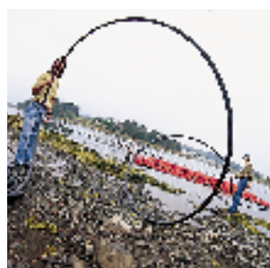
The installation of a sea water based heat pump system
