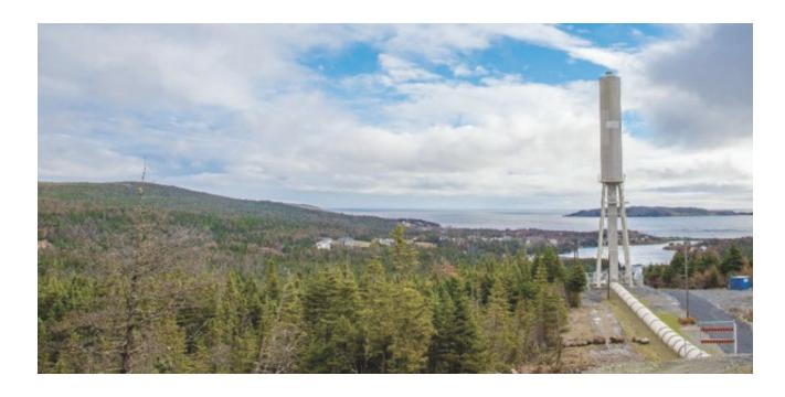
Newfoundland Power's Pierre's Brook hydroelectric plant, located in Witless Bay, has been providing reliable energy production for 85 years. Annually, the facility generates approximately 25 GWh of electricity. In 2016, Newfoundland Power invested \$15 million to upgrade the facility to ensure optimal performance for years to come. Other capital programs focus on runner replacements to increase the efficiency of Newfoundland Power's other hydroelectric plants.
